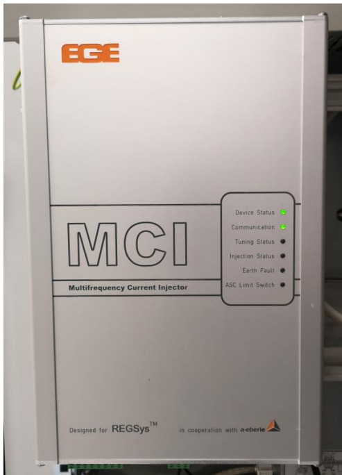
Figure 4: MCI connected to REG-DP(A) with Device Status and Communication LED lit
