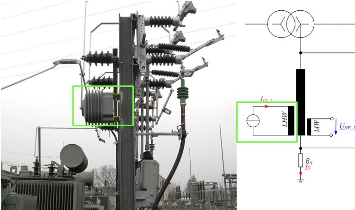
Figure 24: Spare power auxiliary winding (PAW) for current injection
