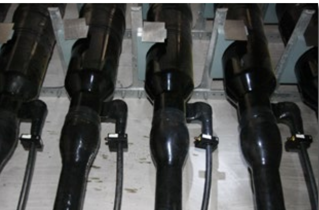
HFCT installation on SECTIONALIZED CABLE JOINTS, around ground connection cables outside link-box.
