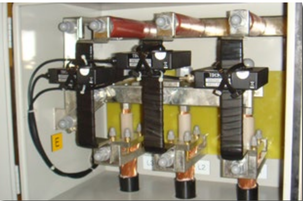
HFCT installation on SECTIONALIZED CABLE JOINTS, around ground connection cables inside link-box.
